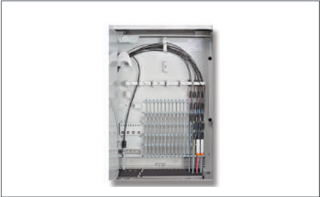
KVZ Street Cabinet Cable Area
